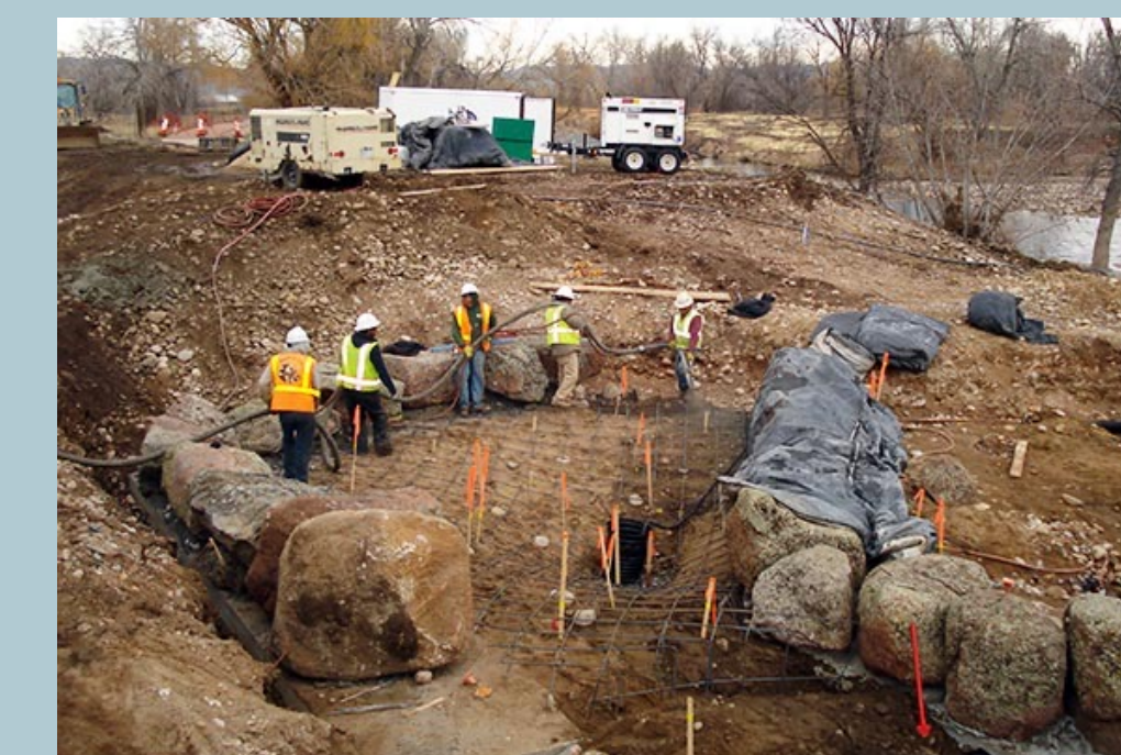
Figure 6: Rehabilitation of West Vine Basin in Fort Collins, CO. 9
