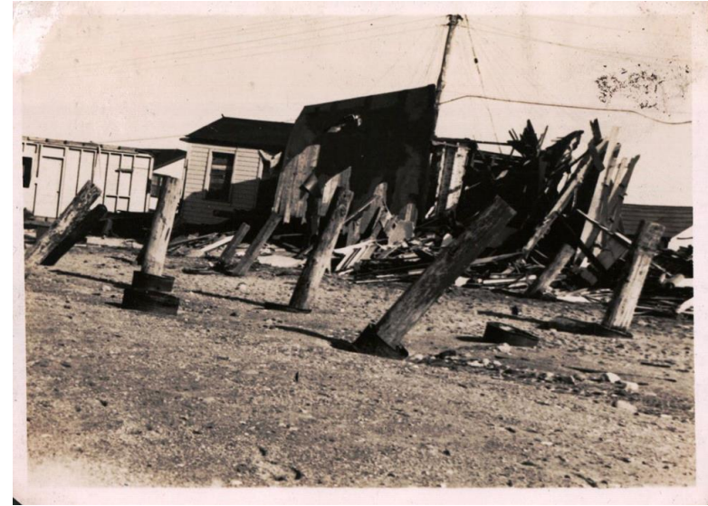
Long Beach West after the 1938 Hurricane (Ref. Town of Stratford)
