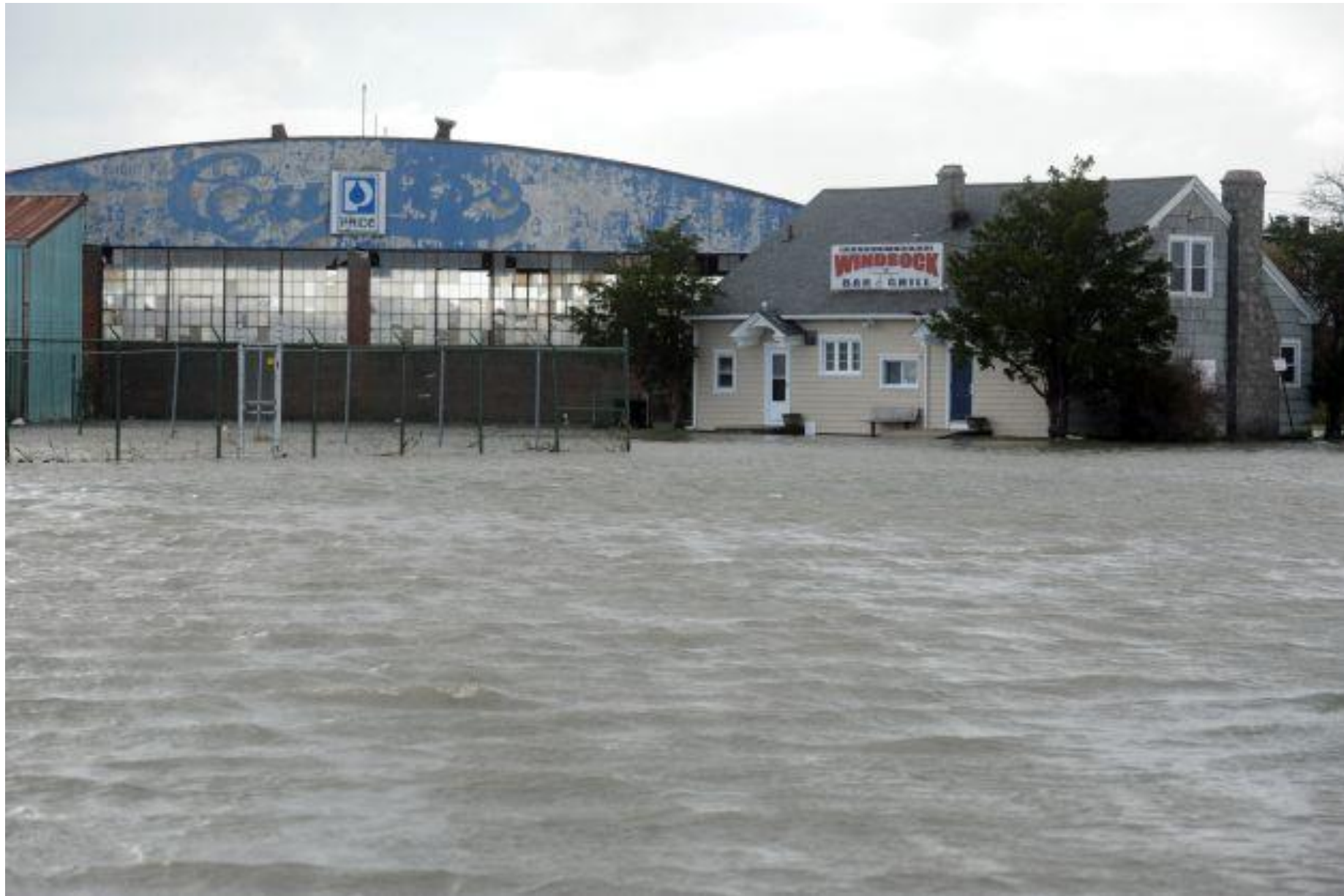
Damaged fuel station at Sikorsky Airport after Sandy (Source: image from ctpost.com)
