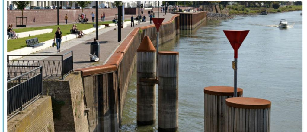
Elevated promenades provide public access to the shoreline and are raised to the Design Flood Elevation (DFE) level to protect inland communities from coastal flooding.
