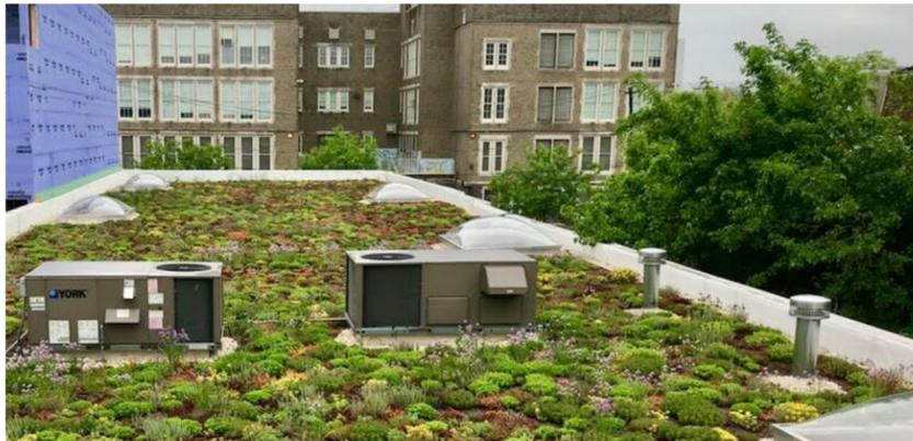
A green roof is a layer of growing medium for vegetation installed over a waterproofing system, slowing down runoff by retaining rainwater and gradually releasing it back into the atmosphere through condensation and transpiration. Blue roofs provide temporary water storage systems that allow for the gradual release or evaporation of stored water.
