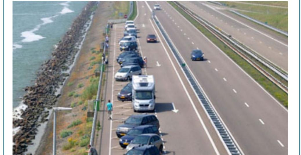
Elevating roadways to target DFE keeps transportation infrastructure dry during the flood events, maintaining evacuation routes and access for emergency services. Elevated roadways may also act as flood protection for inland communities.
