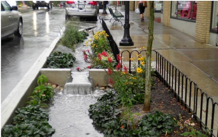
Right-of-way bioswales are vegetated drainage courses located in sidewalks to capture, detain, and infiltrate runoff from streets, allowing any excess rainwater to enter the piped stormwater system.
