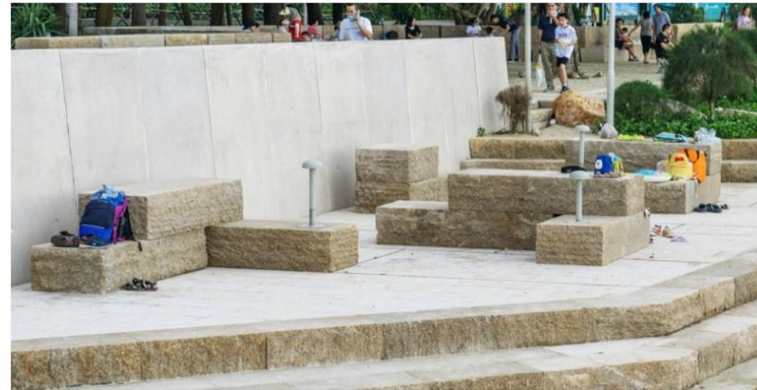
Bulkheads are concrete structures along shorelines of large bodies of water that protect from flooding, wave action and erosion. Elevated bulkheads can be integrated into recreational greenways and provide waterfront access to users.
