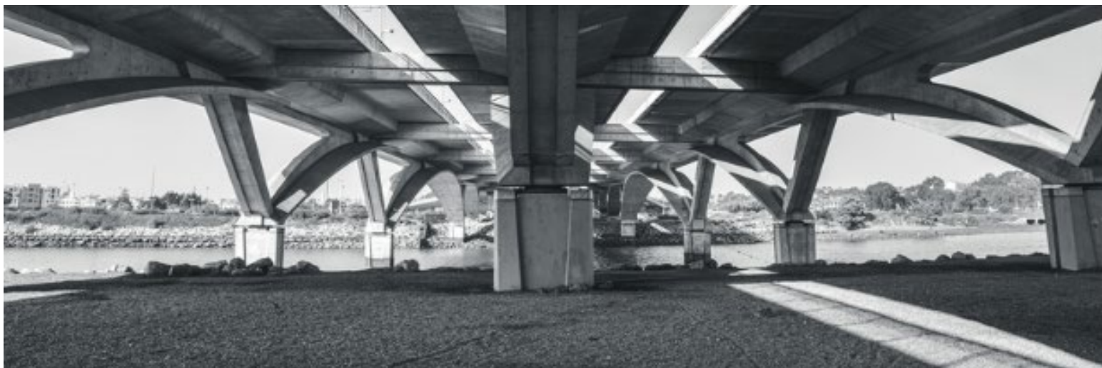
View from under Bridge in Bridgeport, CT (free image: Canva).
