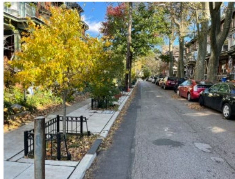
Use of stormwater tree trenches in Phila., PA
