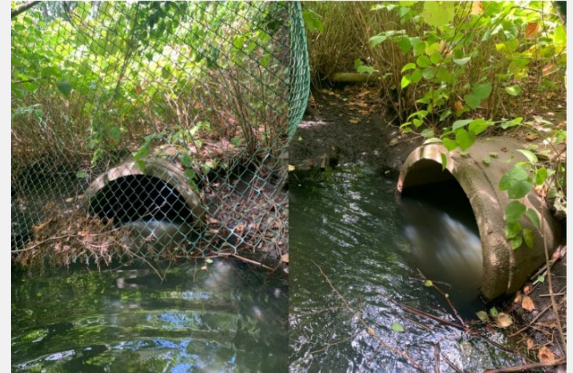
Image of the 48" Mill Plain Road Outfall Pipe (Image credit: SLR, 2022)
