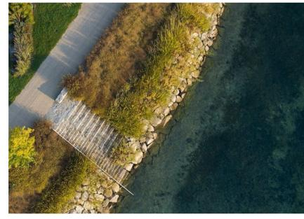
Revetments are hard sloping structures, typically constructed using natural stone, or concrete blocks designed to reduce shoreline erosion by absorbing wave energy and minimizing wave run-up. Sometimes these structured systems are necessary and can be altered as hybrid systems to incorporate ecological features providing enhanced habitat opportunities as well as enhance quality of life and water quality.
