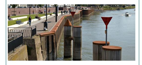
Elevated promenades provide public access to the shoreline and are raised to the Design Flood Elevation (DFE) level to protect inland communities from coastal flooding.
