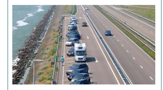
Elevating roadways to target DFE keeps transportation infrastructure dry during the flood events, maintaining evacuation routes and access for emergency services.
