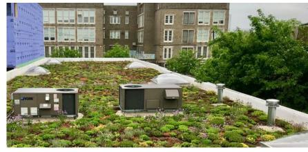
A green roof is a layer of growing medium for vegetation installed over a waterproofing system, slowing down runoff by retaining rainwater and gradually releasing it back into the atmosphere through condensation and transpiration. Blue roofs provide temporary water storage systems that allow for the gradual release or evaporation of stored water.
