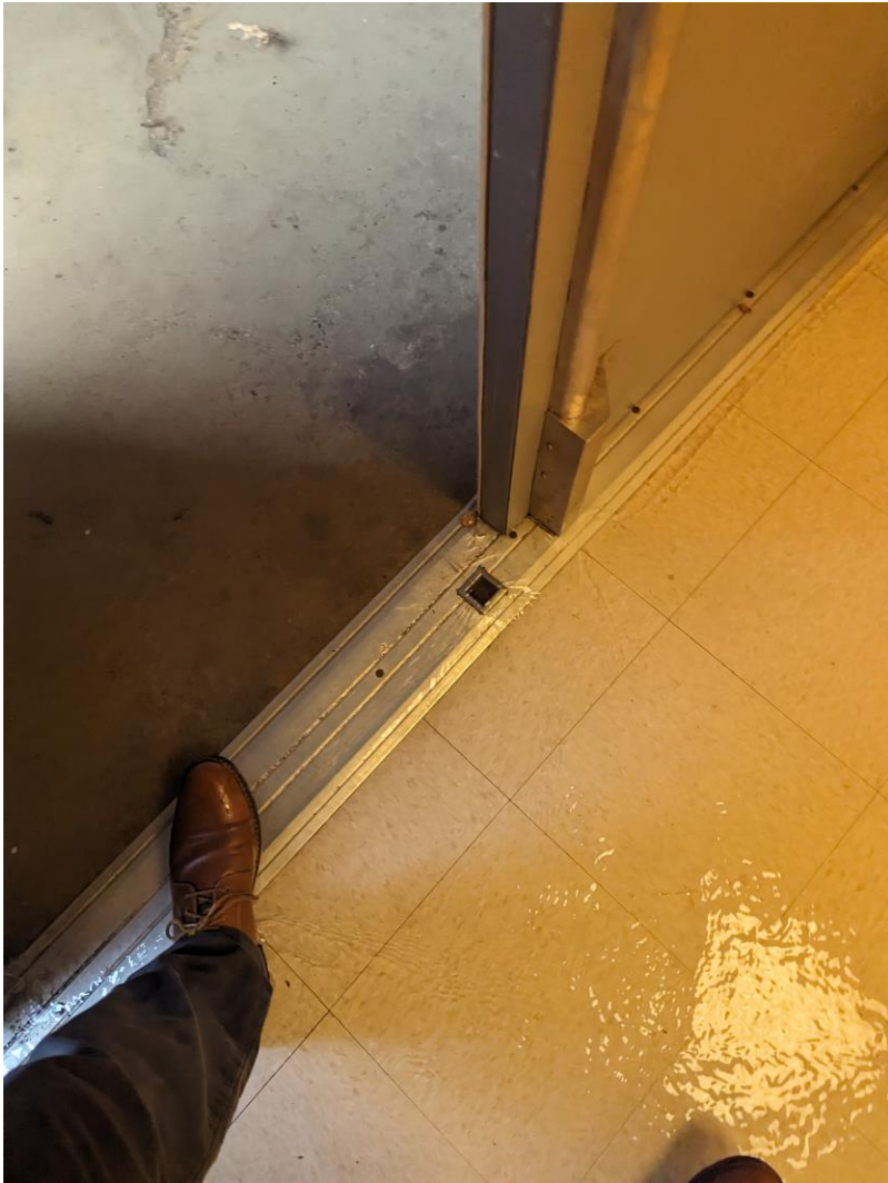
Senior Center Basement, September 2023
