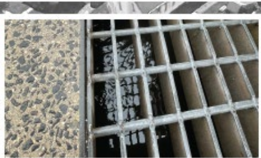
2 Standing Water in Catch Basins | Catch basins in the parking lot were observed with standing water.
