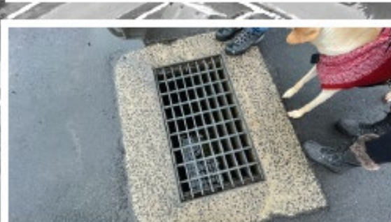
2 Standing Water in Catch Basins | Catch basins in the parking lot were observed with standing water.
