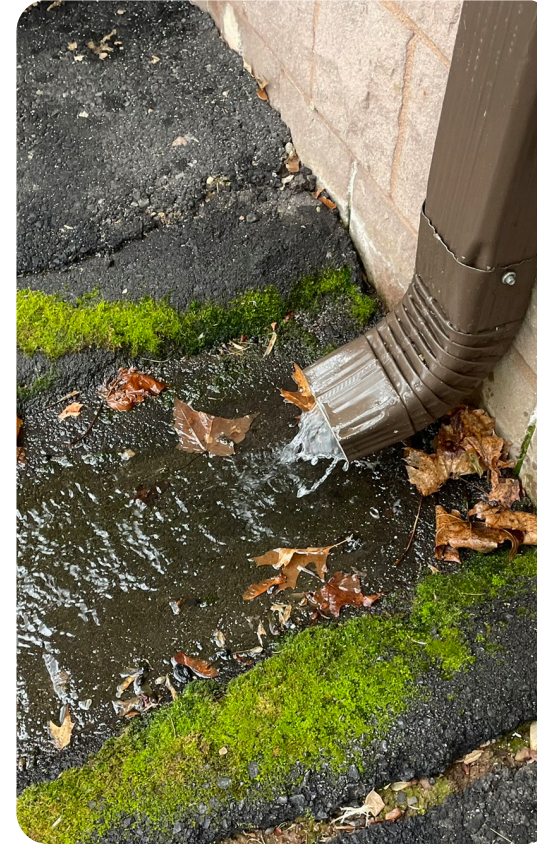
Image of Portland Library roof drainage taken during first site visit
