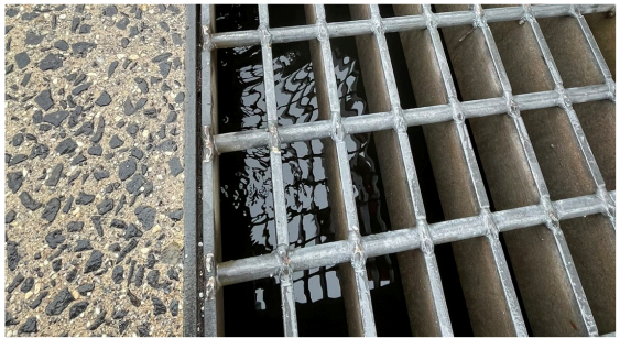
2 Standing Water in Catch Basins | Catch basins in the parking lot were observed with standing water.
