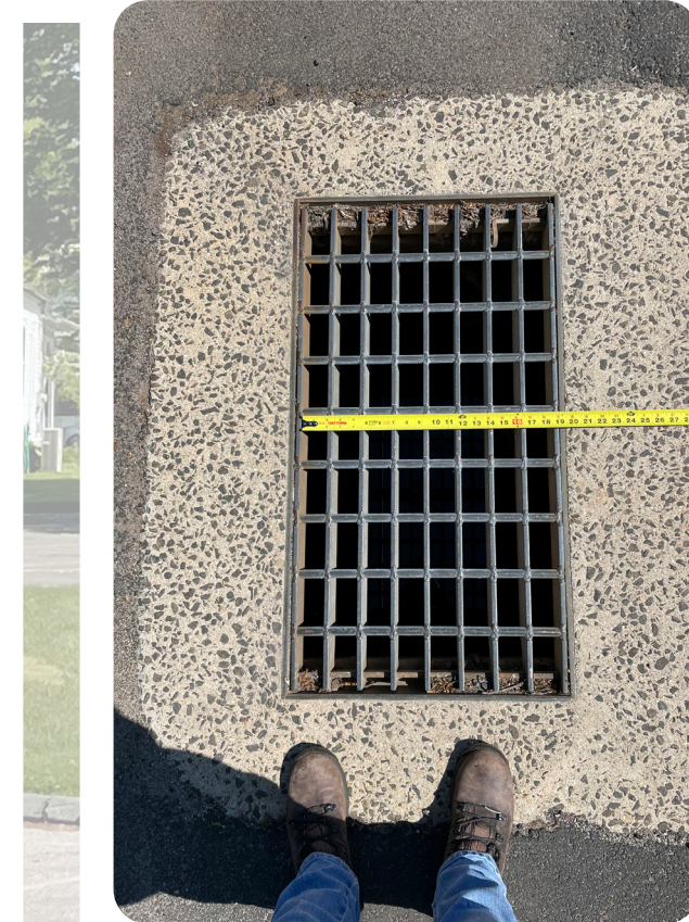
Image of catch basin analysis needed for modelling purposes, which was performed during second site visit
