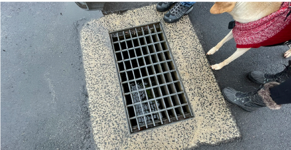
2 Standing Water in Catch Basins | Catch basins in the parking lot were observed with standing water.
