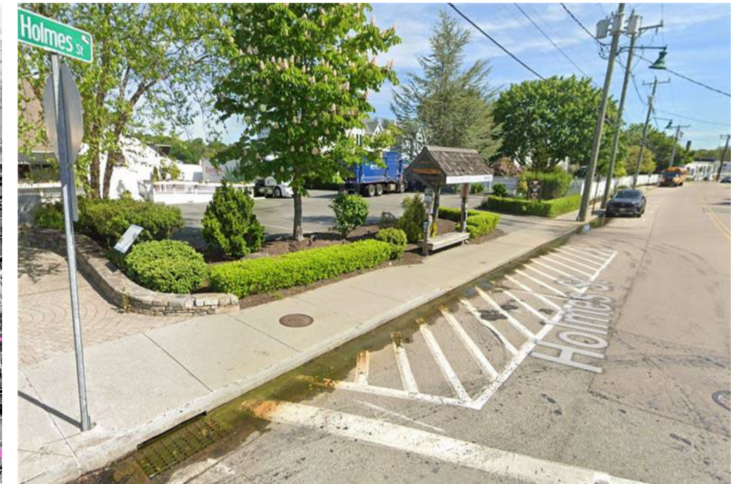
Holmes Street catch basin showing signs of backflow from the Mystic River (Google Streetview)
