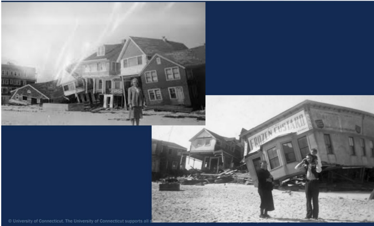
Figure 35. Impacts from the Great Hurricane of 1938 on Ocean Beach (New London, CT) Source: University of Connecticut, Center for Land Use Education and Research
