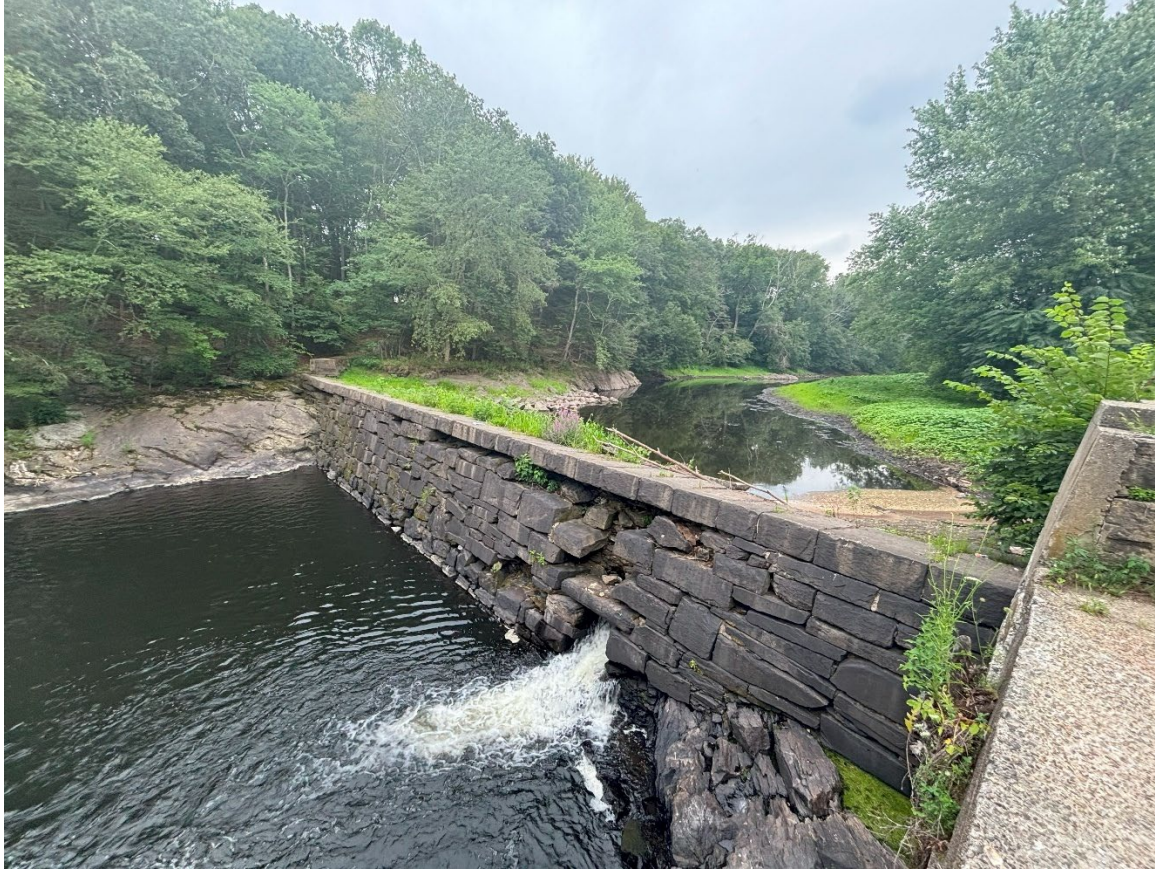
Figure 29. Falls Mill Upper Dam
