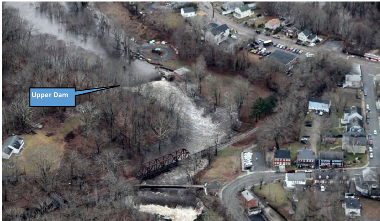
Figure 28: Falls Mill Upper Dam during January 2024 Flood (Photo Credit: CT Division of Emergency Management and Homeland Security)
