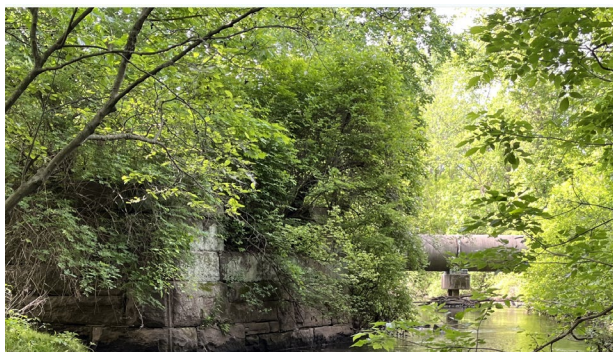
Figure 26: Old railroad abutment/embankment and existing sewer line
