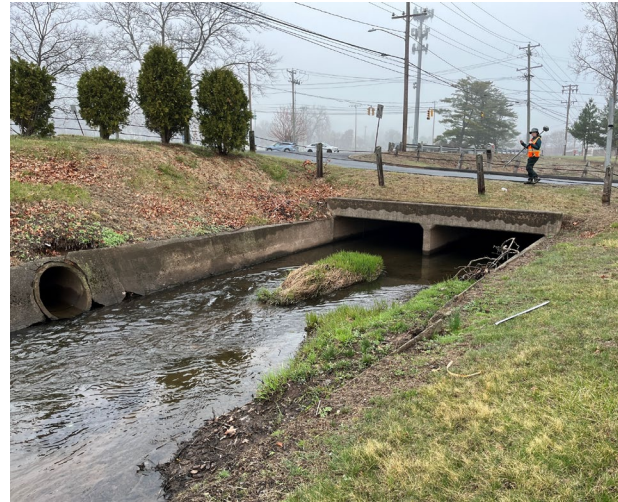
Figure 14: Twin box culverts at Xtreme Rides
