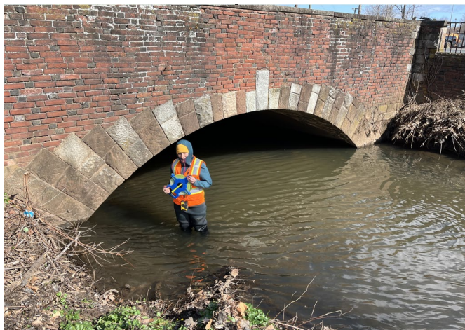
Figure 21: Existing arch bridge at Veterans Stadium Willow Brook Park
