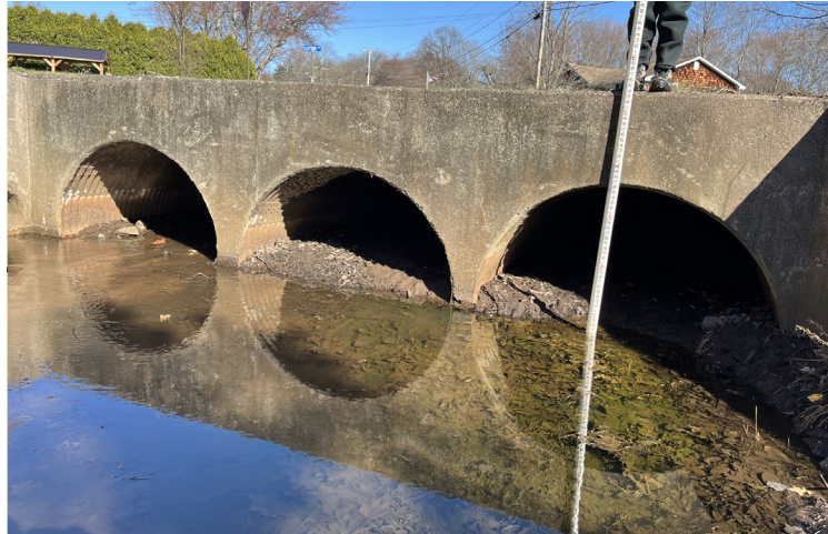
Figure 9: Existing three-barrel pipe arch culvert at Coles Avenue
