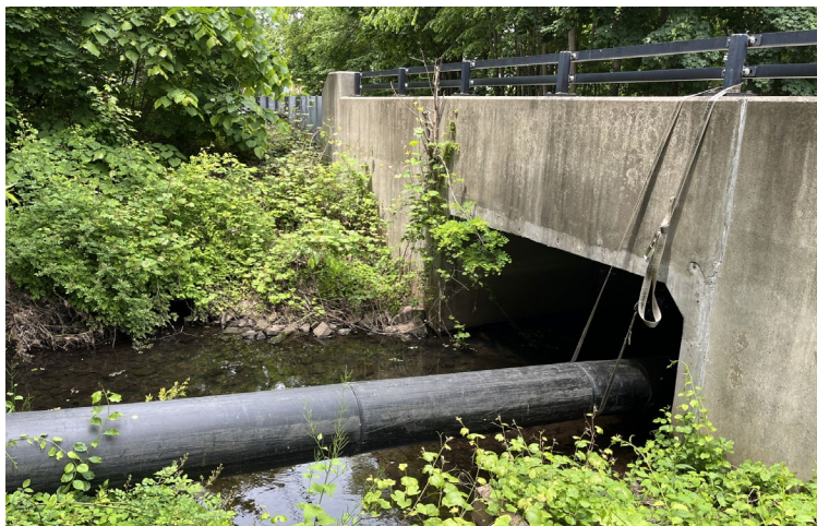
Figure 5: Existing bridge at Wilson Avenue
