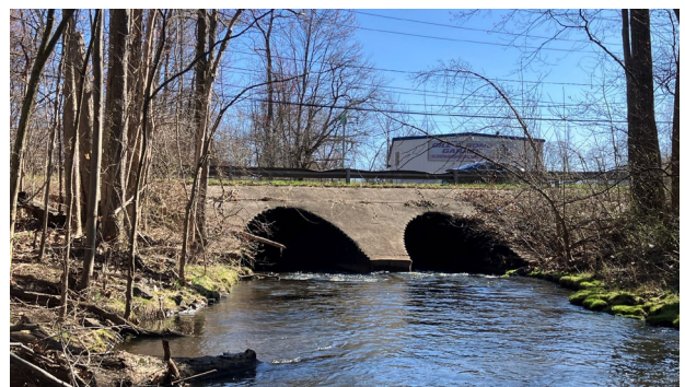
Figure 25: Existing two-barrel culvert
