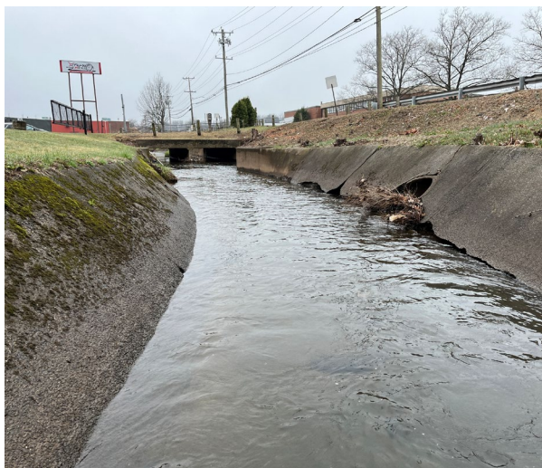
Figure 13: Hardened channel at Xtreme Rides
