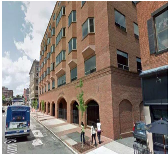
370 Asylum street, an adaptive reuse of a former office building in downtown Hartford. ©Google Maps 2026
